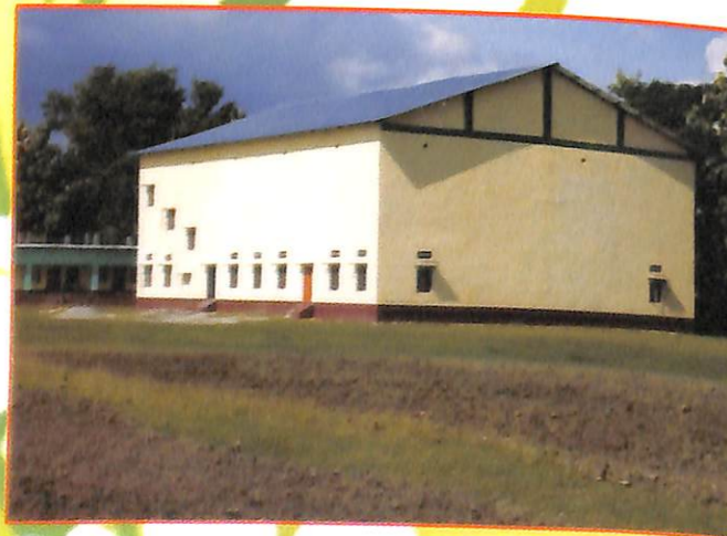
In-door Sports Complex
